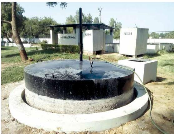
**Picture 2: Dairy Effluent Scum-Based Biogas Plant at M/S Vidya Dairy, Anand**
