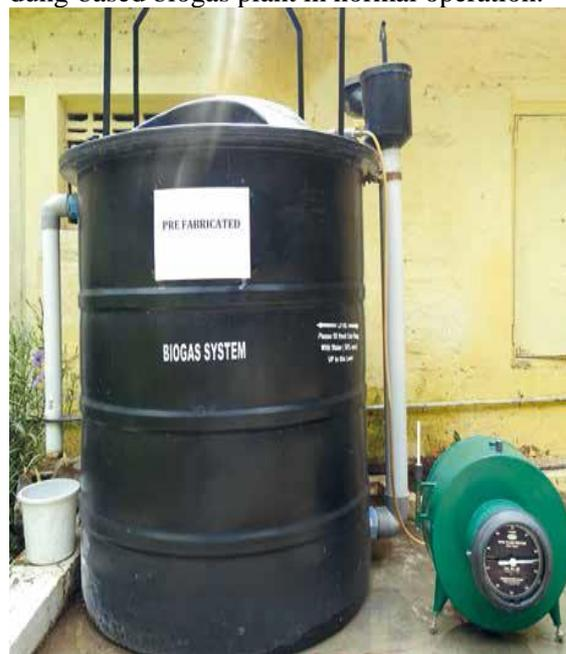
**Picture 1: Pictorial View of a 900 L Capacity Biogas Plant**
